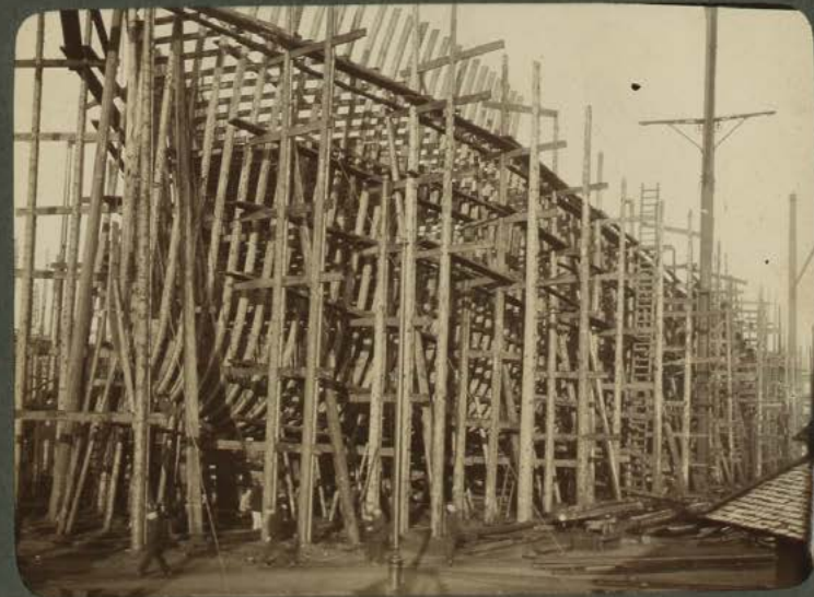
761 - Aug 1 - Finished Framing Top of Stem Not Up Yet.
